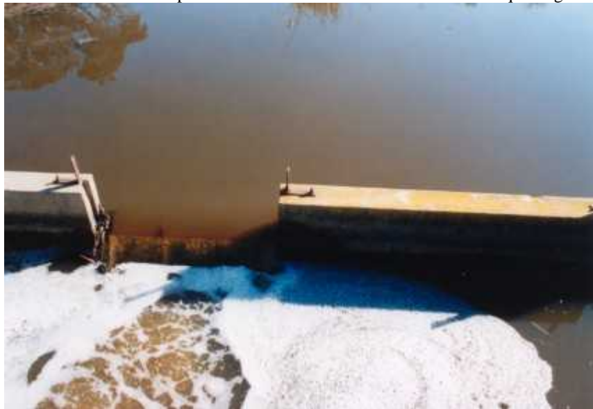
This small structure protects Mcleods Morass from salt water intrusion.
